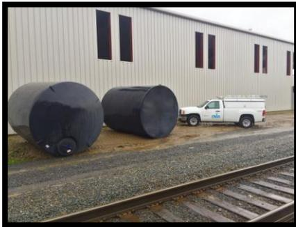
**End Result:** The three rainwater systems reduce the overall impact of the peak flow of runoff from the new commercial building
